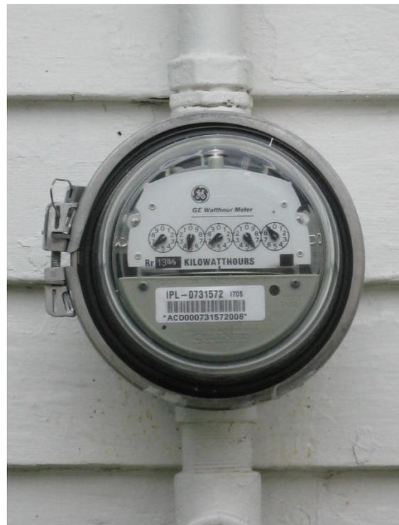
Figure 2 – typical 60A S-Base meter
