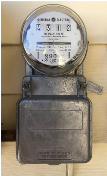
Figure 1 – self-contained A-Base meter
